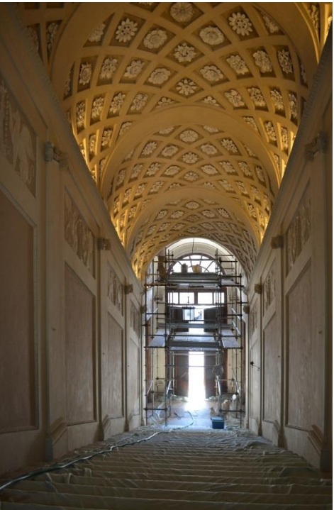
Restoration of surfaces
